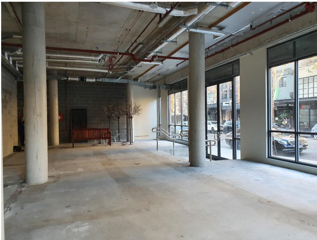
Figure 4: Site viewed internally looking north (accessible toilet in north-western corner)
