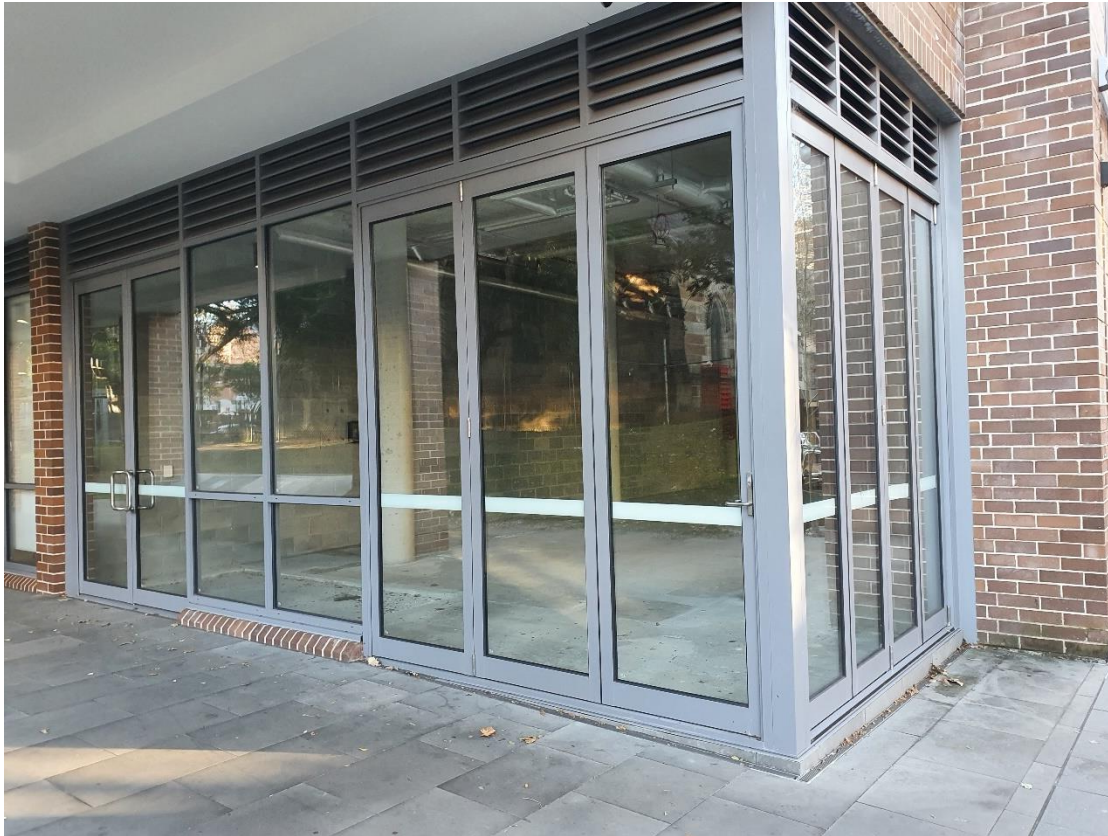
Figure 3: Subject tenancy viewed from St Johns Church pedestrian link looking north-west
